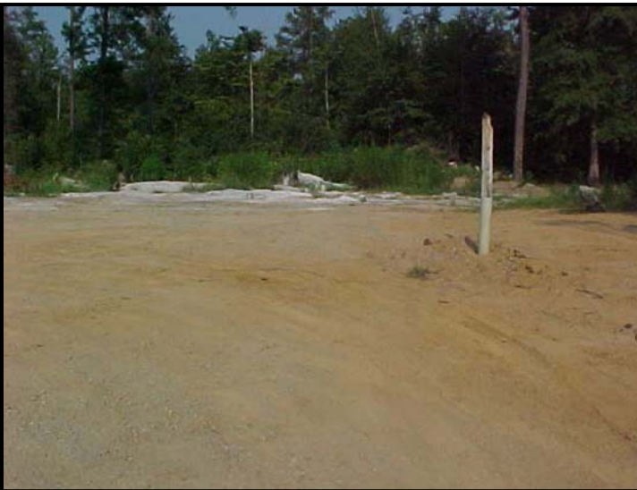
Looking at Phase 2 from end of Myers Creek Dr.
